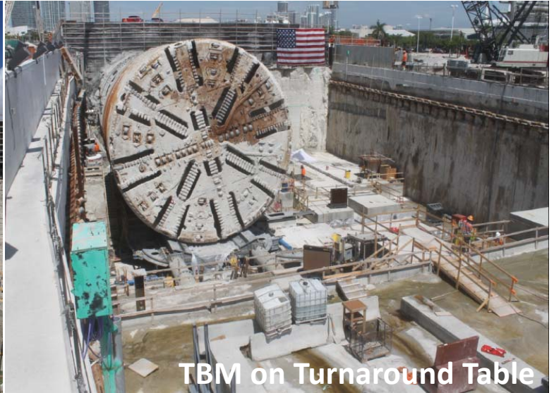
TBM Breakout
