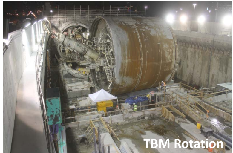
TBM on Turnaround Table
